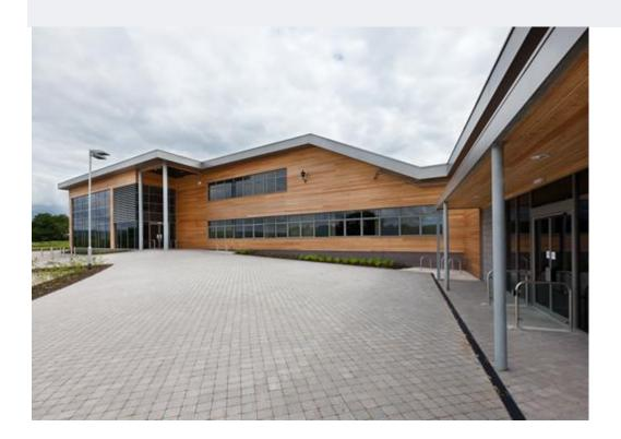
Joint Services facility combining Police station, Fire station and Magistrates' Court. The contractor, John Weaver Construction Ltd required a bespoke and easy to install soffit, fascia and coping system, whilst the client required a durable and aesthetically pleasing system in the same RAL 9007 colour as the windows and doors. Alutec's bespoke composite aluminium system met their requirements perfectly.
